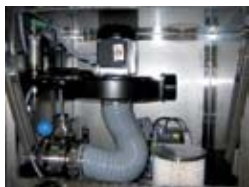
Blower with speed control and HEPA filter for the transfer chamber
